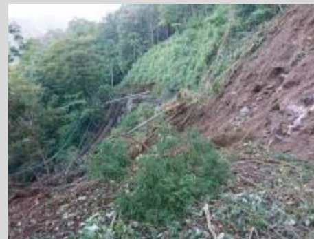
Slope failure
