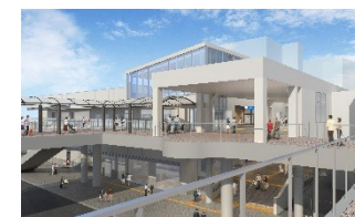
Fujisawa Station (Scheduled for completion in FY2027)
