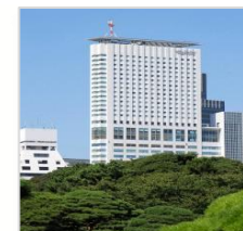
Odakyu Southern Tower
