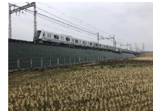
Repair embankment slopes in order to control damage, including from landslides
