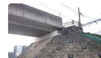
Seismic reinforcement (Sakai River)
