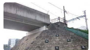
Seismic reinforcement (Sakai River)
