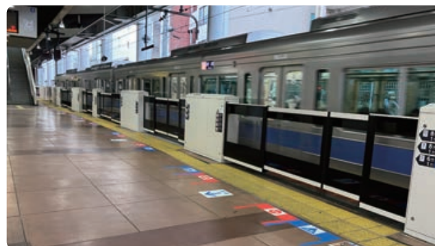
Platform doors at Sagami-Ono Station
